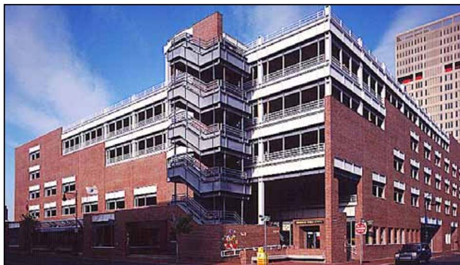
East Cambridge parking garage
